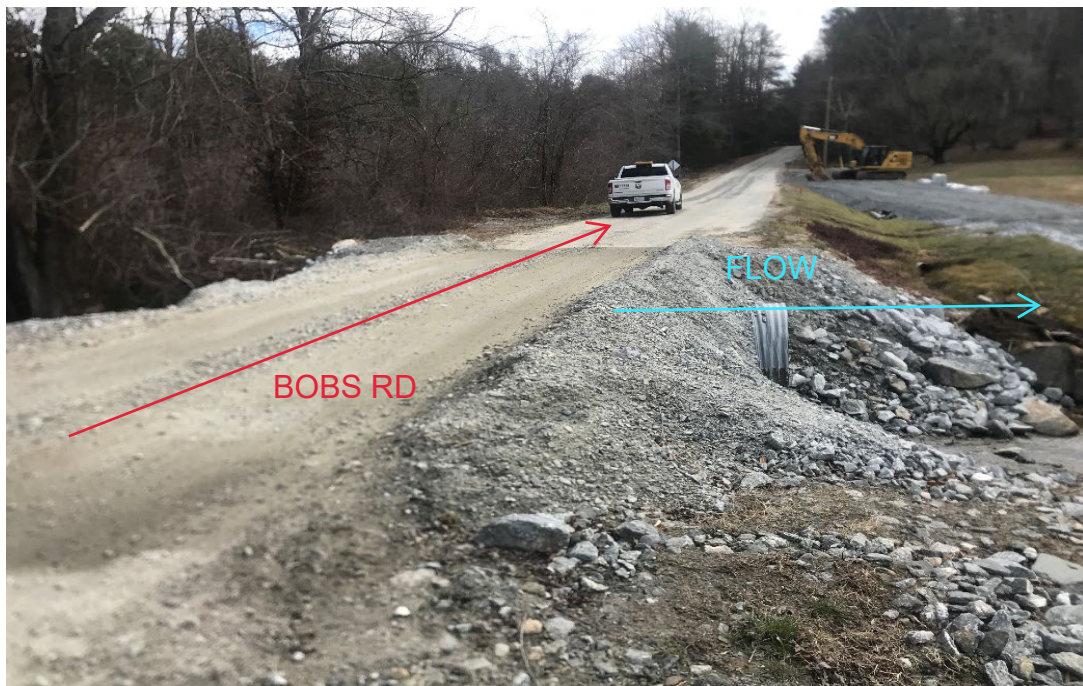
Figure 2-View to East from End Bent 1 towards End Bent 2 on downstream side
