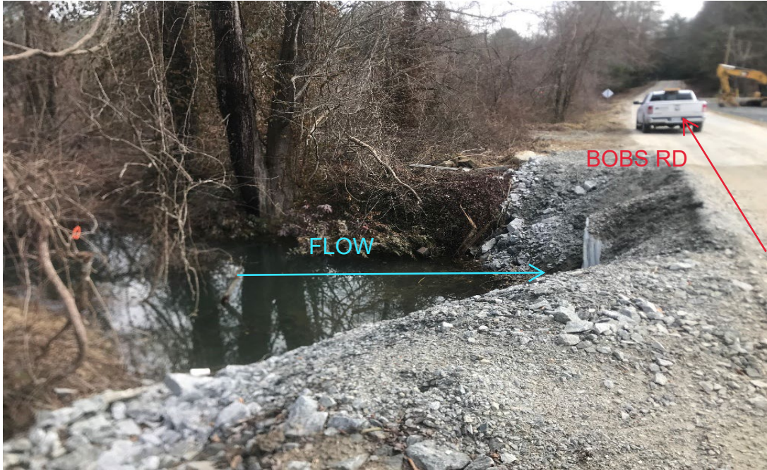
Figure 1-View to East from End Bent 1 towards End Bent 2 on upstream side
